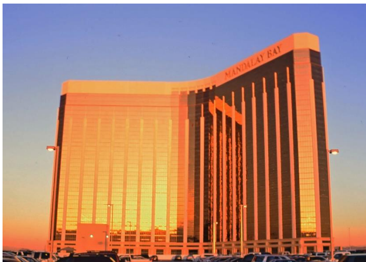
Figure 1. Gold-coated windows of Mandalay Bay Casino-Hotel, Las Vegas, reflecting the setting sun. Photo by Samuel Pellicori.
